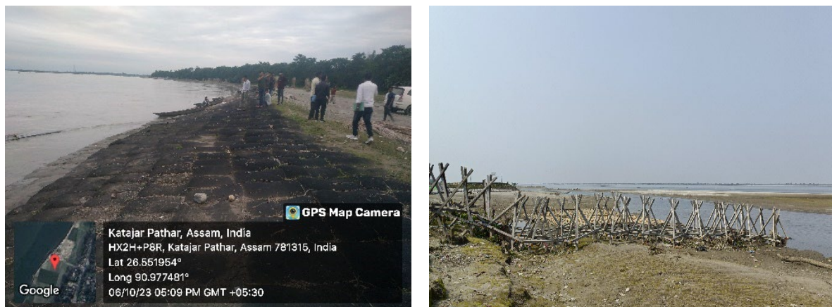
Figure 2-5: Photographs of typical anti-erosion and Porcupine works.
