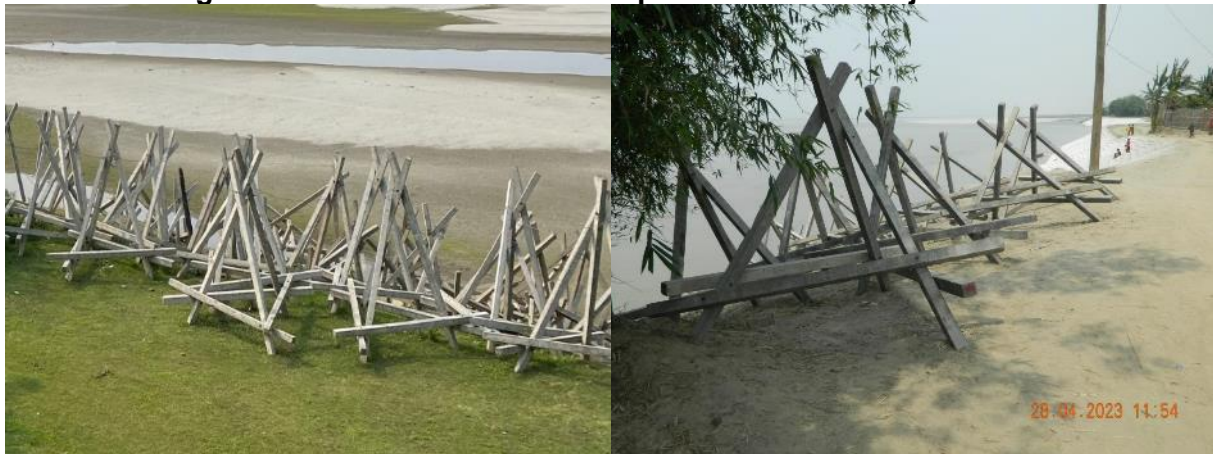
Figure 2-8: Presence of old Porcupine screens in Project Area 14
