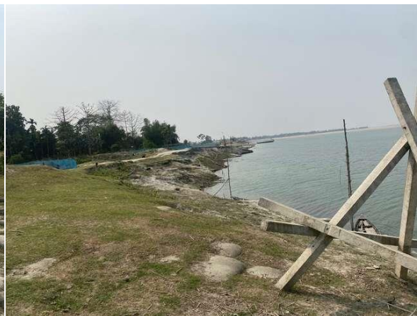
Proposed site for anti-erosion and flood protection works at Lotordia
