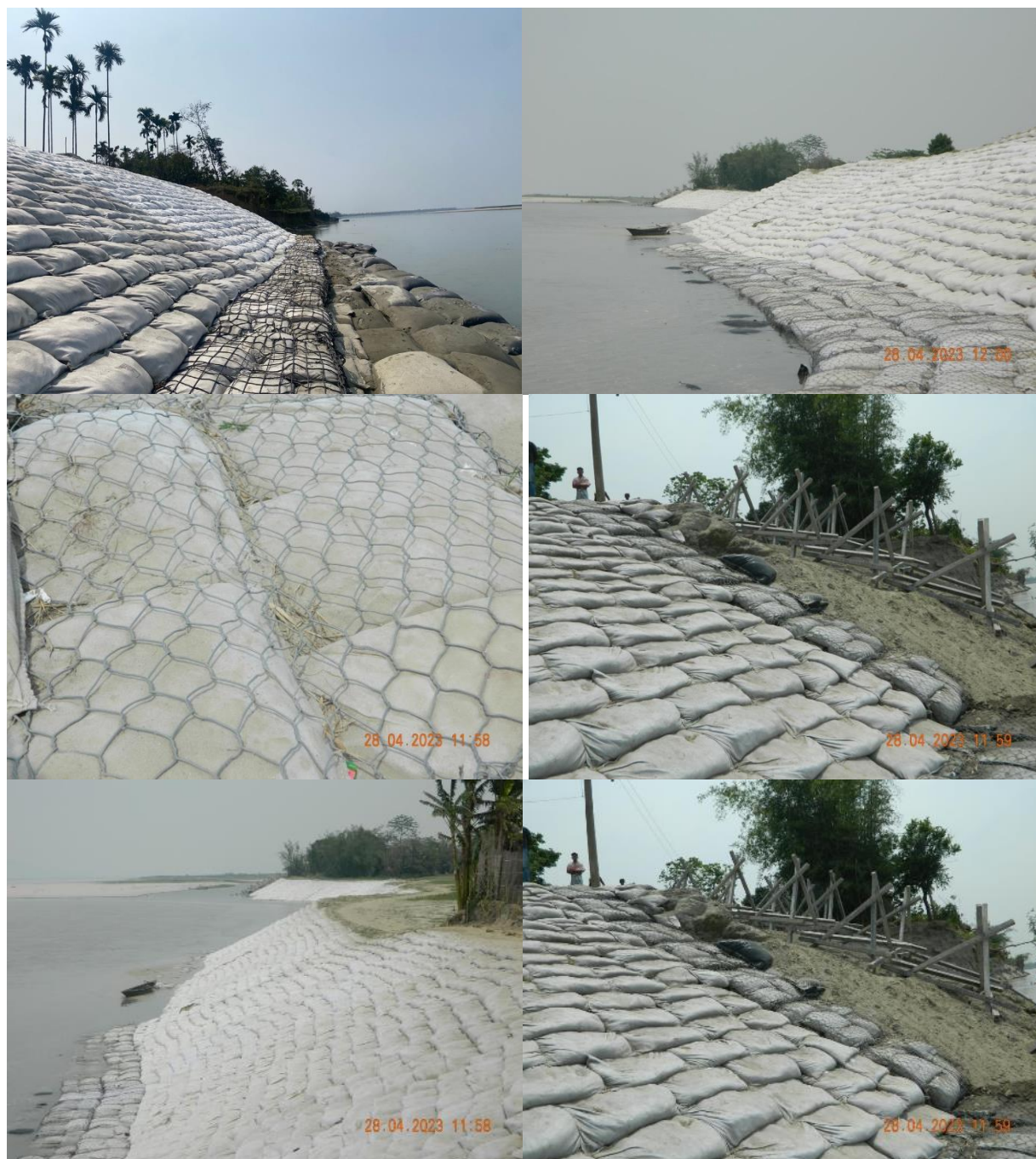
Figure 2-7: Use of Geo textile bags for Anti erosion works 13
