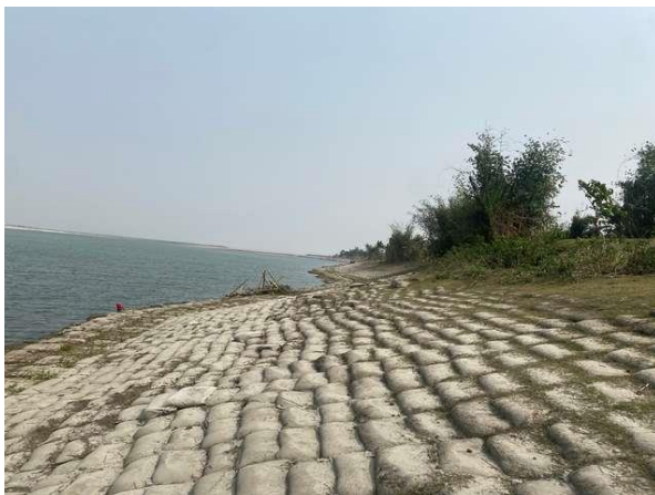
Upstream/downstream AE & FB work done by WRD/Assam Government at Lotordia
