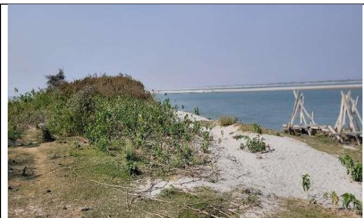
Growth of Grasses along the Protection Work
