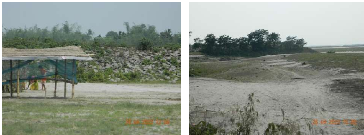
Start of subproject interventions stretch n Laharighat area (Mikirgaon - Kathani - Tengaguri area)
