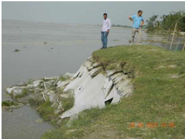
Erosion of existing AE works in Balidunga – Baralimari area
