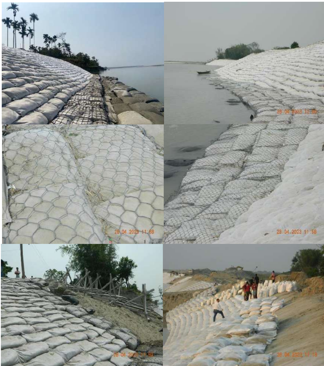
Figure 2-5: Use of Geo textile bags for Existing AE works 11
