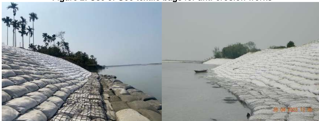
Figure 2: Use of Geo textile bags for anti-erosion works
