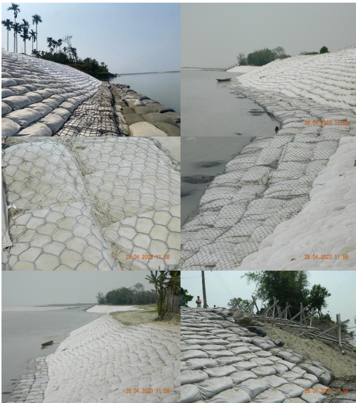
Figure 2-7: Use of Geo textile bags for Existing AE works 12
