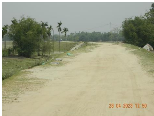
Existing Embankment in Chunari to Jaleswar area
