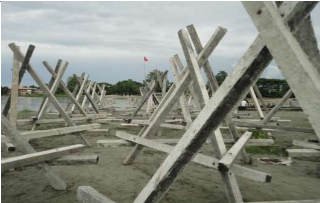
Figure 6: Typical anti-erosion work with CC block revetment and geobag apron (Motholla AE works at Motholla area by WRD)
