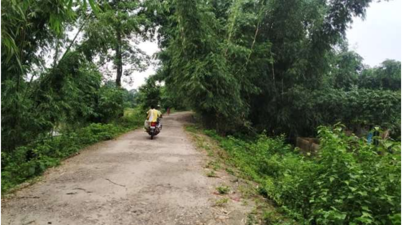
Figure 9 Existing condition of the Embankment at Chunbari (Lot-1)
