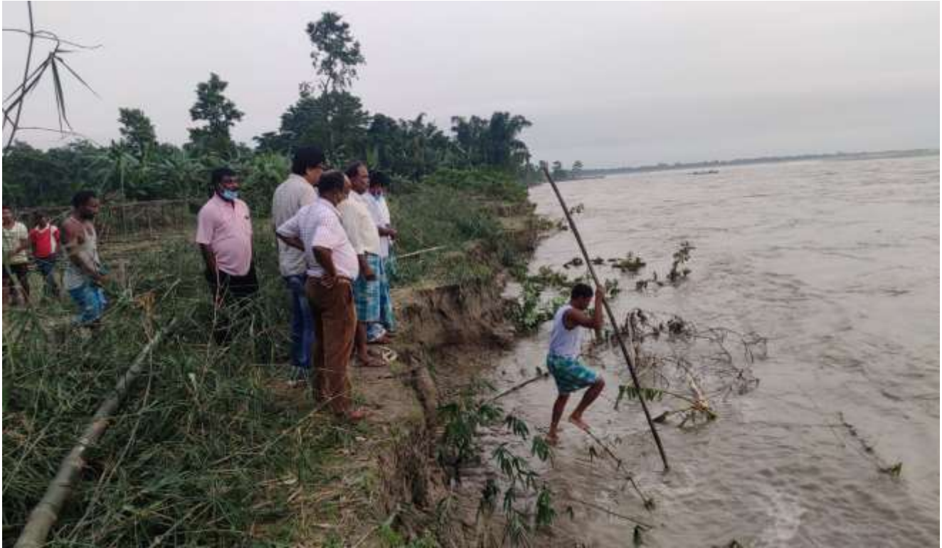
Figure 7 Erosion at Elengbari
