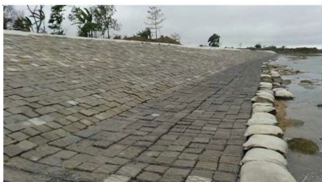
(b) CC Block Revetment with Geobags
