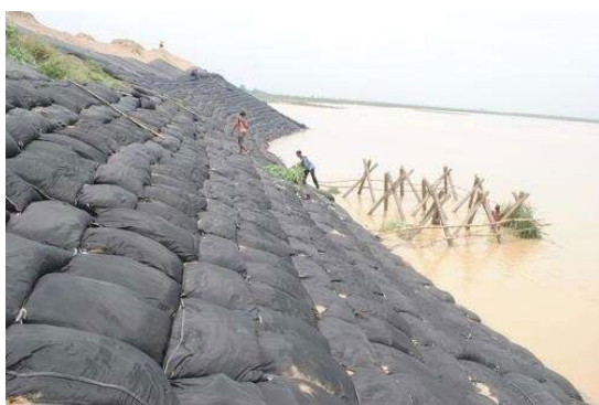
(a) Revetment with Geobags
