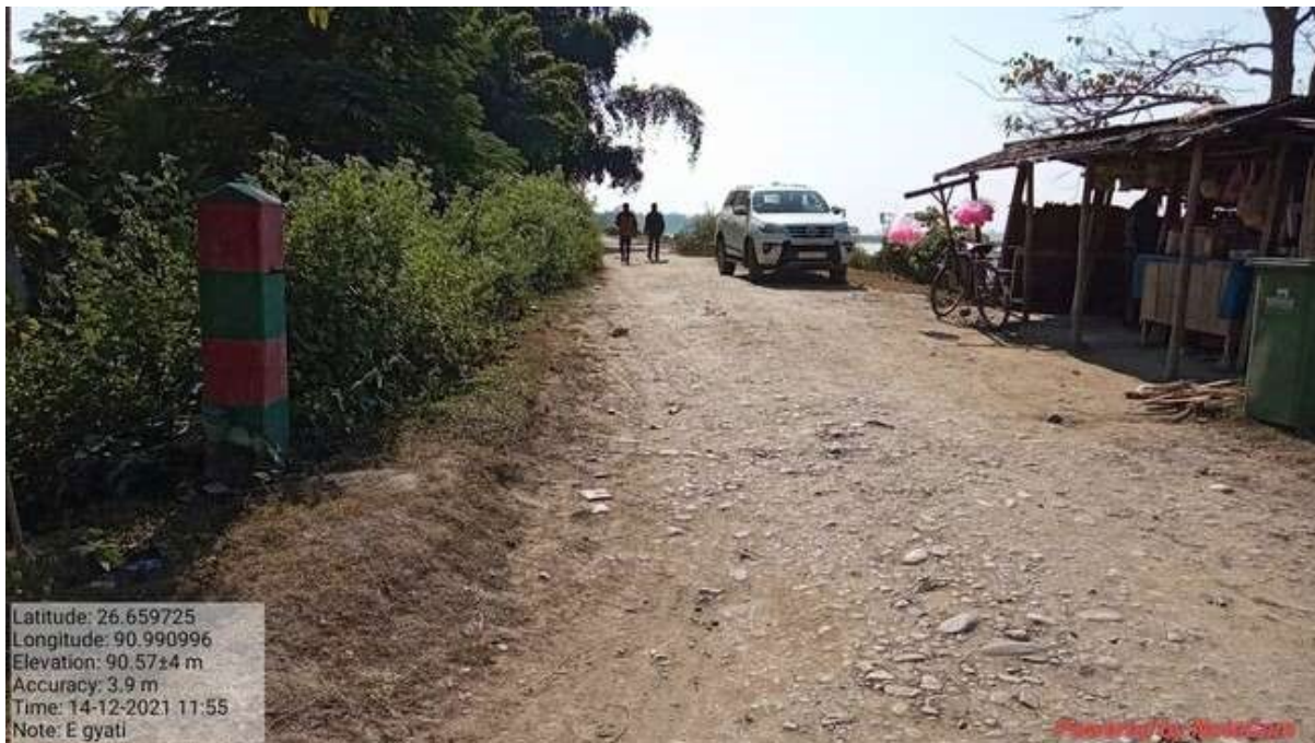
Figure 2: Current Condition of Embankment (R/S-1)
