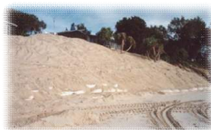
Figure 4-13: Bank after implementation of geo-bags
