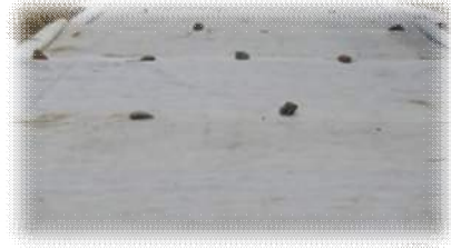
Figure 8-3: Geo-textile laid out on rolled surface
