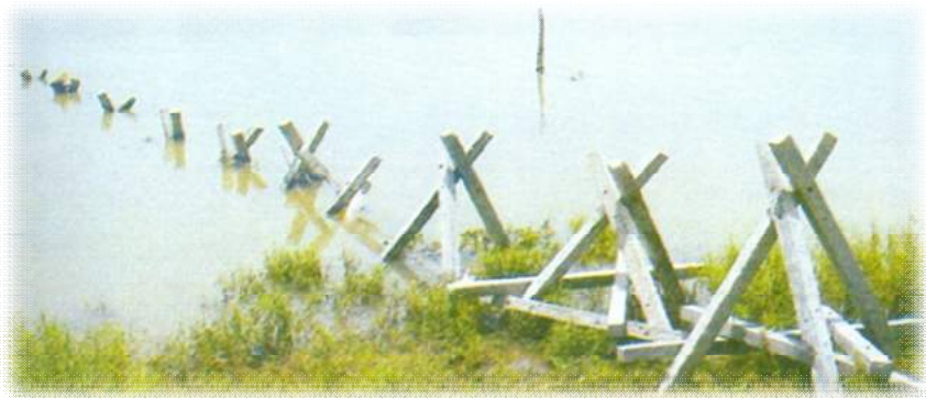
Figure 6-2: Typical RCC porcupine screen
