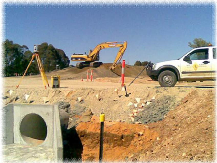
Figure 7-2: cross drain under the embankment
