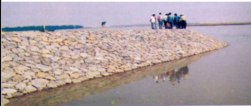
Figure 5-1: Spur built with boulders
