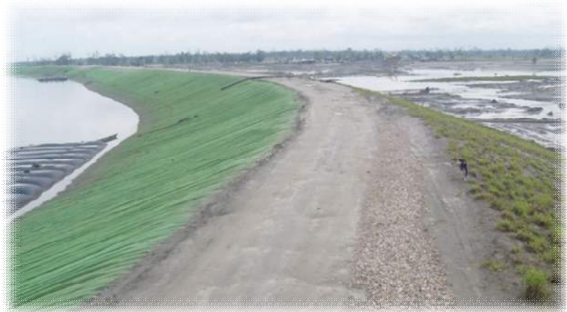
Figure 3-9: A typical completed embankment with R/S slope protection with mattress and turfing on C/S slope and road on crest
