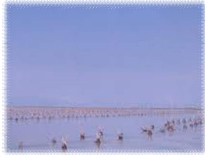
Figure 6-1: RCC porcupines for slackening the flow
