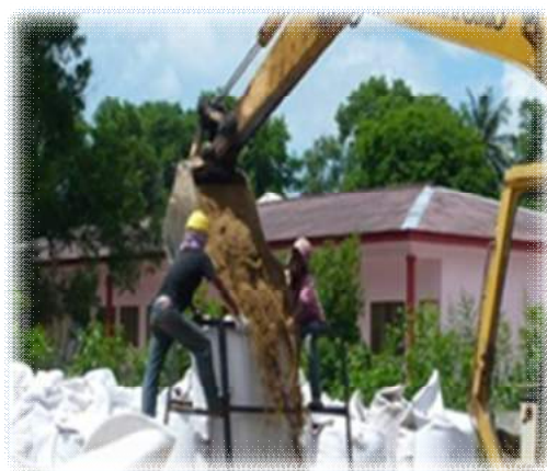
Figure 8-11: Filling of geo-bags
