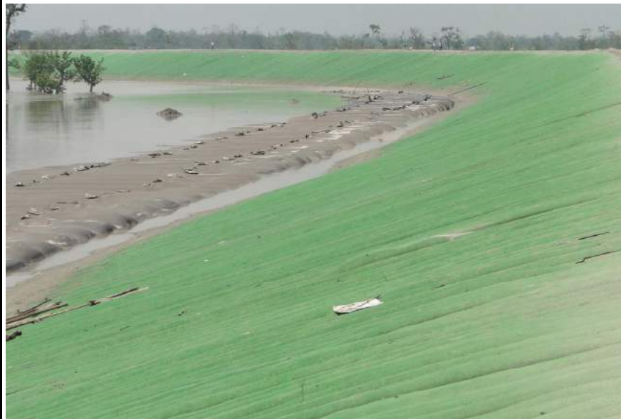
Figure 3-1: Typical high embankment with slope protection using sand filled geo-matress
