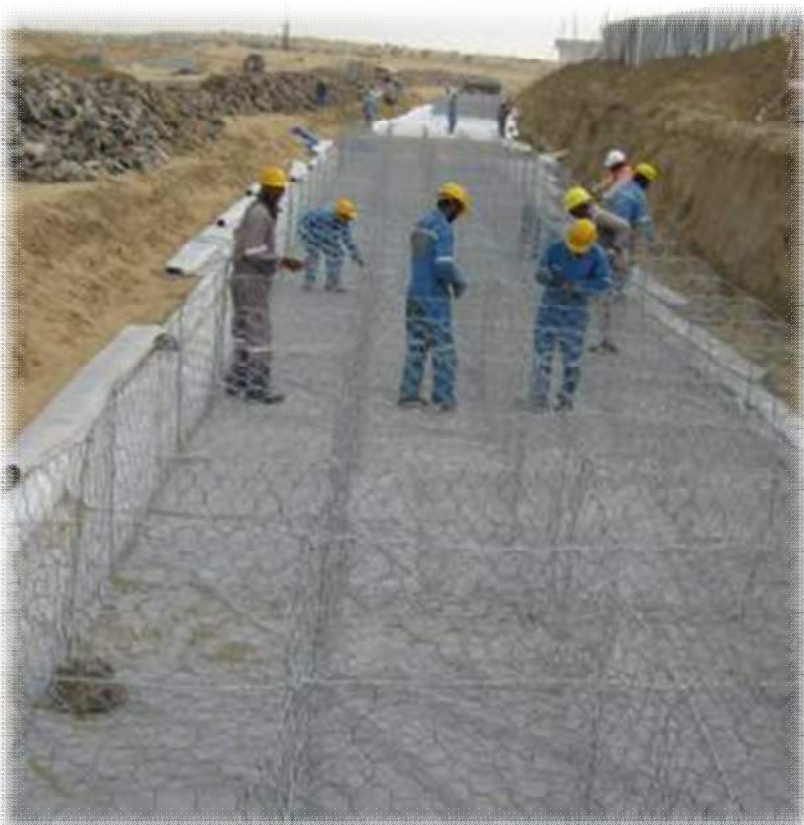
Figure 8-6: Laying and connecting all adjacent gabions
