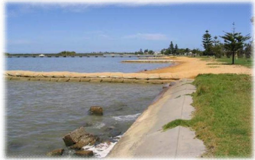
Figure 5-7: Spur along with bank protection using geo-textile
