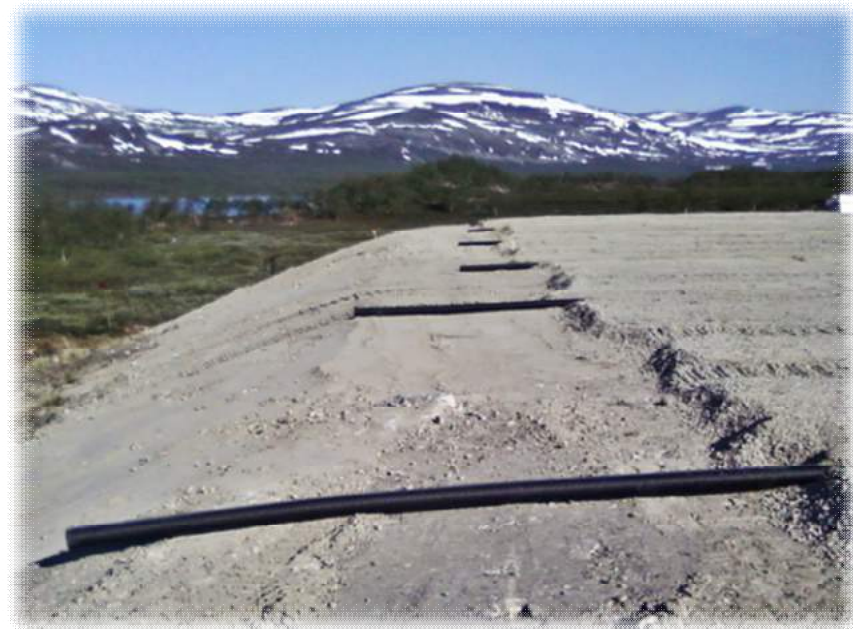
Figure 3-7: Provision of drain pipe
