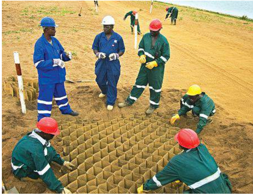
Figure 4-7: A typical Neoweb® preparation
