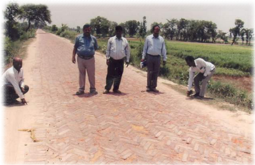
Figure 3-4: An embankment crest with brick soling
