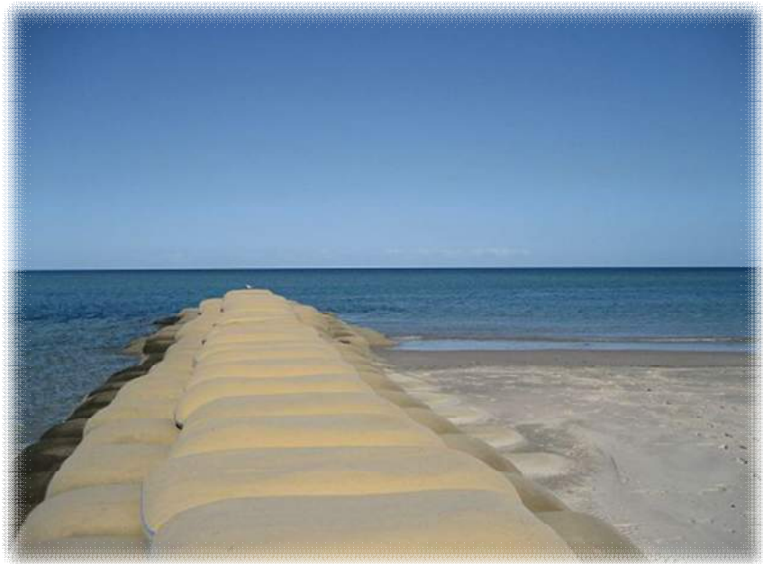
Figure 5-6: Spur using geo-bags
