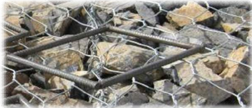
Figure 8-8: Boulders filled in gabions
