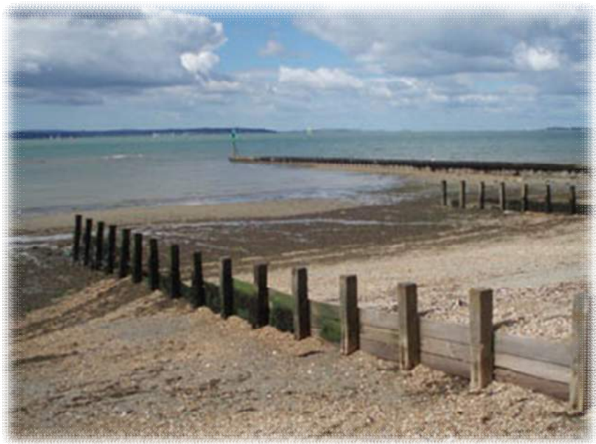
Figure 5-3: Permeable spurs constructed with timber
