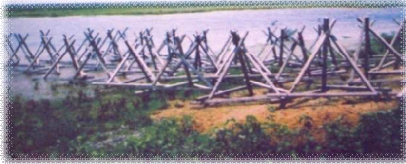
Figure 6-4: RCC porcupine spur
