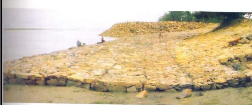
Figure 4-8: A typical bank pitching in wire crates
