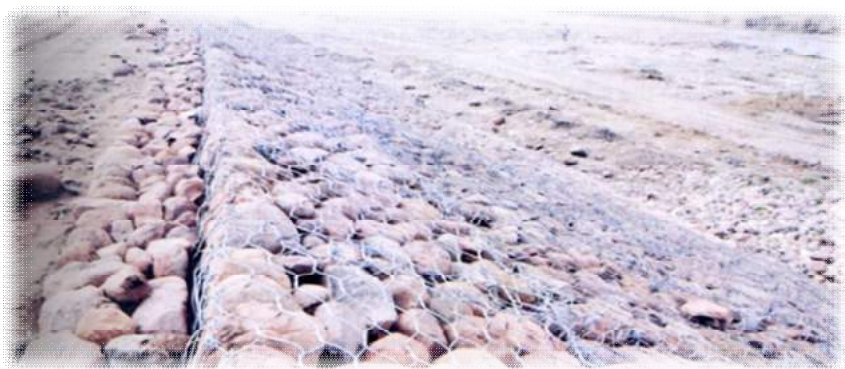
Figure 4-9: A typical bank pitching in crates
