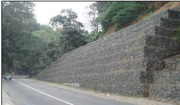
Figure 8-1: Gabion retaining wall
