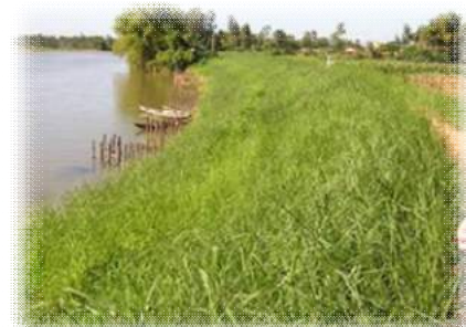
Figure 4-4: Bank after the vetiver implementation
