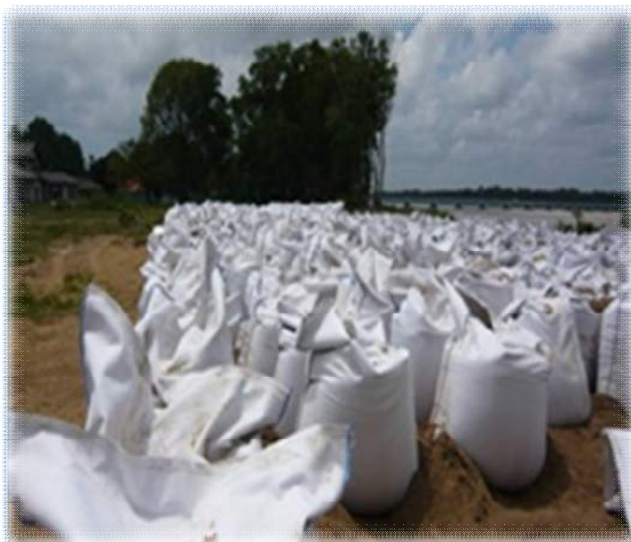
Figure 8-12: Stitching of geo-textile bag
