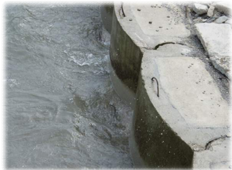
Figure 4-11: Use of cement blocks in bank protection
