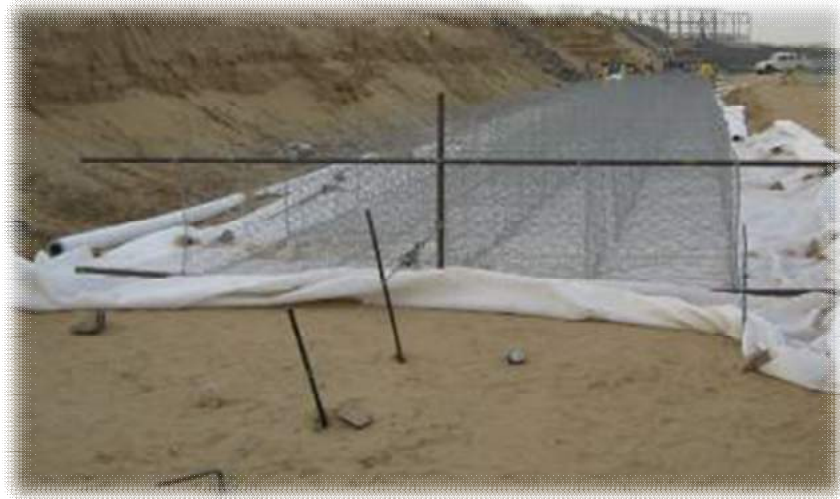
Figure 8-7: Stretching the gabions
